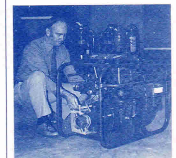
Newly appointed Regional Officer, Murray Sherwell, doing a regular maintenance battery check on a H/Q pump.
